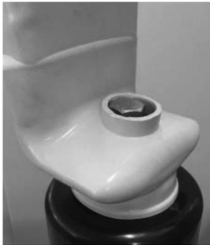
c) screw the bolt M12 with torque  $50 \pm 2$  H\*m and cover the ISM terminal tightly by put insulator CBdet\_RubberIns\_3
