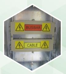
Individually operated earthed metallic shutters are automatically driven during the movement of the VCB from the test to the service position and vice versa. The busbar and cable shutters can be separately padlocked in the open position to prevent accidental contact with any live parts.
