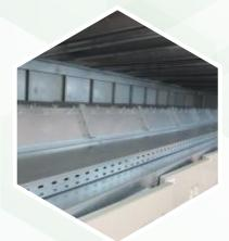
The gas exhaust duct accommodates all three pressure relief flaps and is mounted on the top of each panel. It runs along the whole length of the switchboard. The pressure generated by the internal arc makes a pressure relief flap open thus allowing hot gases to run into a special chimney to be evacuated to dedicated areas.
