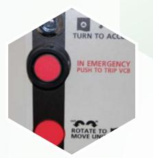
**An emergency trip push-button** is located in the center of the panel. It has a striking, protruding design protected against accidental operation. The trip button can be quickly spotted in an emergency.
