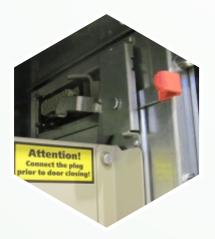
**An LV plug interlock** visually prompts an operator to connect the draw-out unit to secondary circuits before the compartment door is closed.
