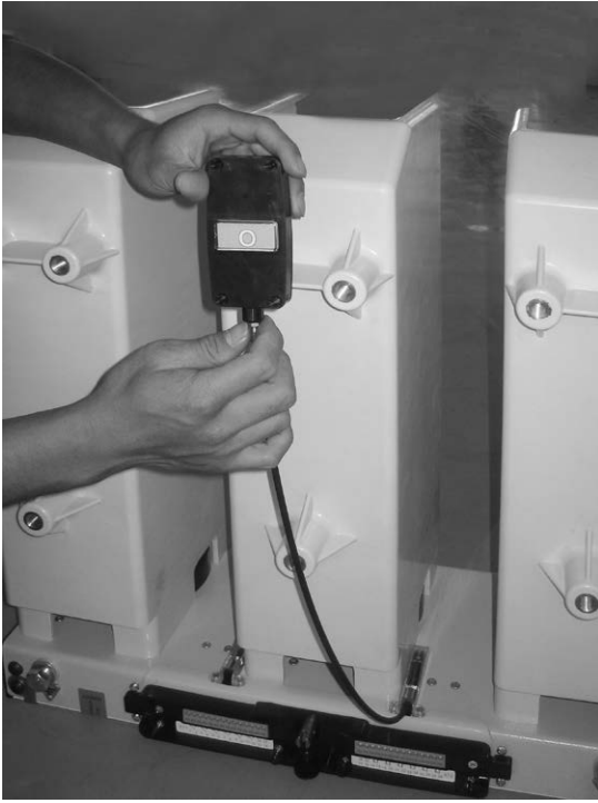
Figure 76 Adjust the indicator for both closed and opened states of the switching module.
