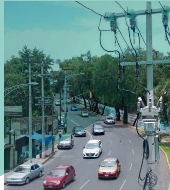
▲ Automatic circuit recloser in the grid automation project in Mexico city
