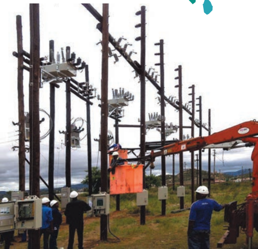
▲ 27 kV outdoor substation with automatic circuit reclosers
