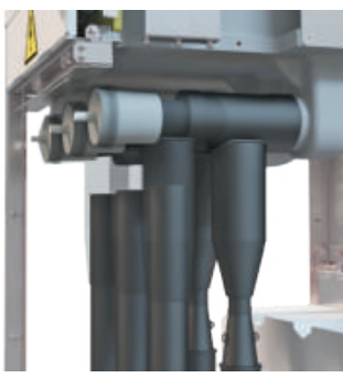
Voltage sensors at T connectors
