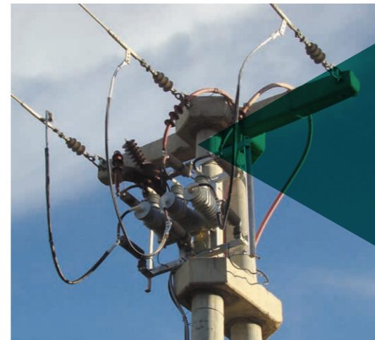
▲ Fuse-switches replacement in Turkey
