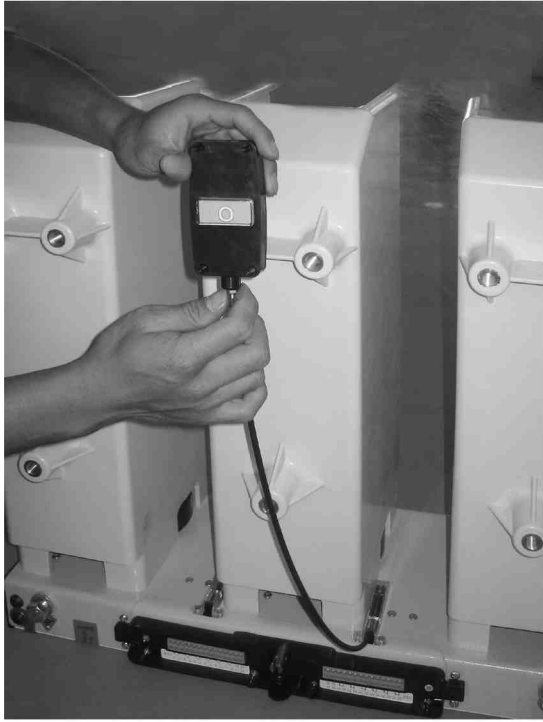
Figure 68 Adjust the indicator for both closed and opened states of the switching module.
