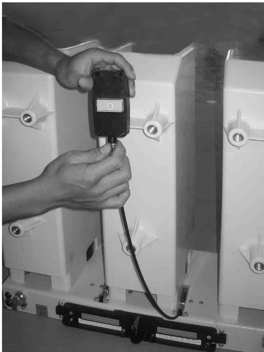
Figure 64 Adjust the indicator for both closed and opened states of the switching module.
